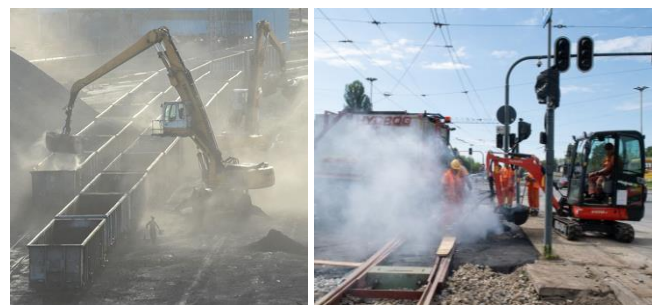
Fig. 1. View of the working conditions of construction machines in the vicinity of the railway and tram tracks [18, 22]
